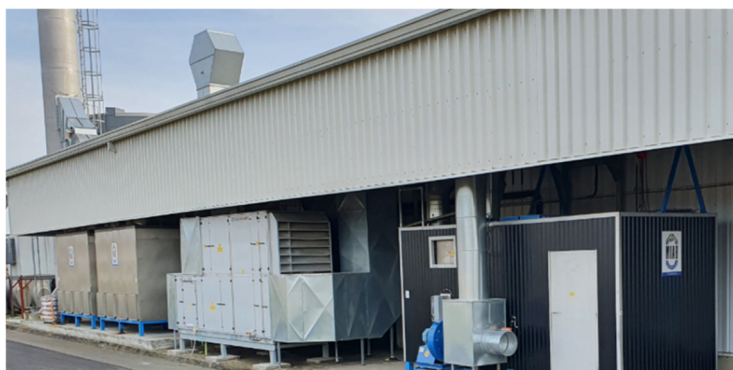
Photo 1. MIAB FD system with two filters, see two stainless steel units to the left, as well as the catalytic oxidization unit, see black unit with a door to the right.
